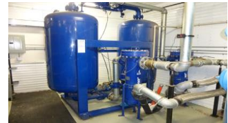
Ar-Tech's Compressor Room produces "quality" air that is dry, and filtered free of oil and contaminants.
