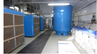
Ar-Tech's Compressor Room produces "quality" air that is dry, and filtered free of oil and contaminants.
