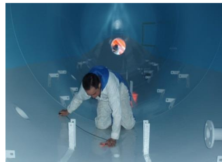
Coating thickness verified through mil checks
