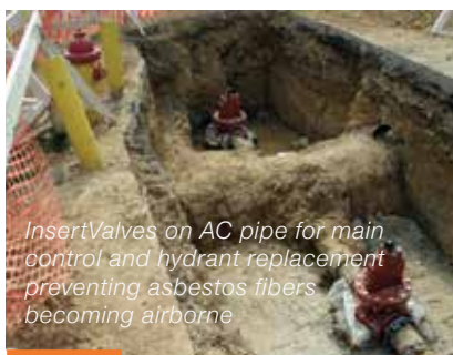
An InsertValve installation under full line pressure.
