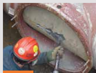
Chipping gun removes mortar
