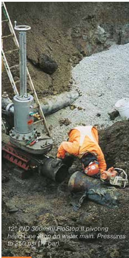
Model IP-142 water main Hot / Wet Tapping machine
