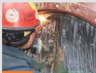
Cutting torch removes reinforcing steel wires
