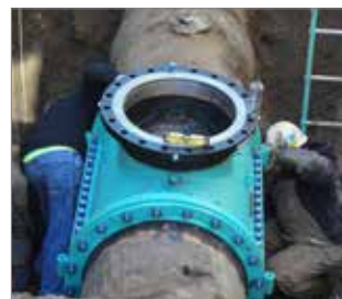
Mechanical joint line-stop fitting installation
