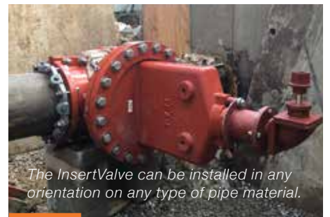
An InsertValve installation under full line pressure.
