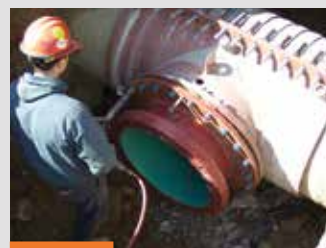
Gland installed and sleeve pressure-tested
