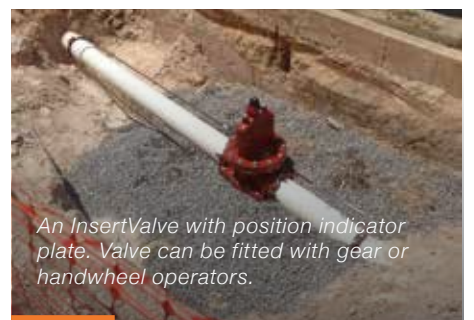
The InsertValve can be installed in any orientation on any type of pipe material.
