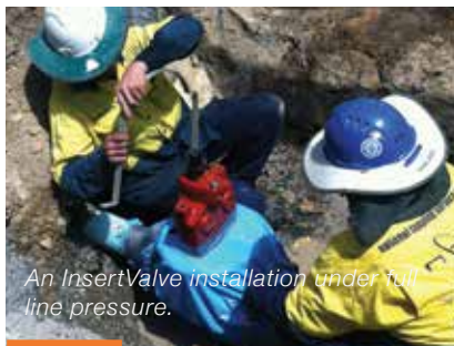
The InsertValve can be installed in any orientation on any type of pipe material.
