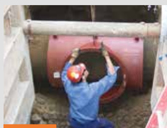
Concrete tapping sleeve mounted
