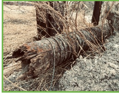
Wooden Stave Pipe Submitted by Scott Baillie, Municipality of Crowsnest Pass
